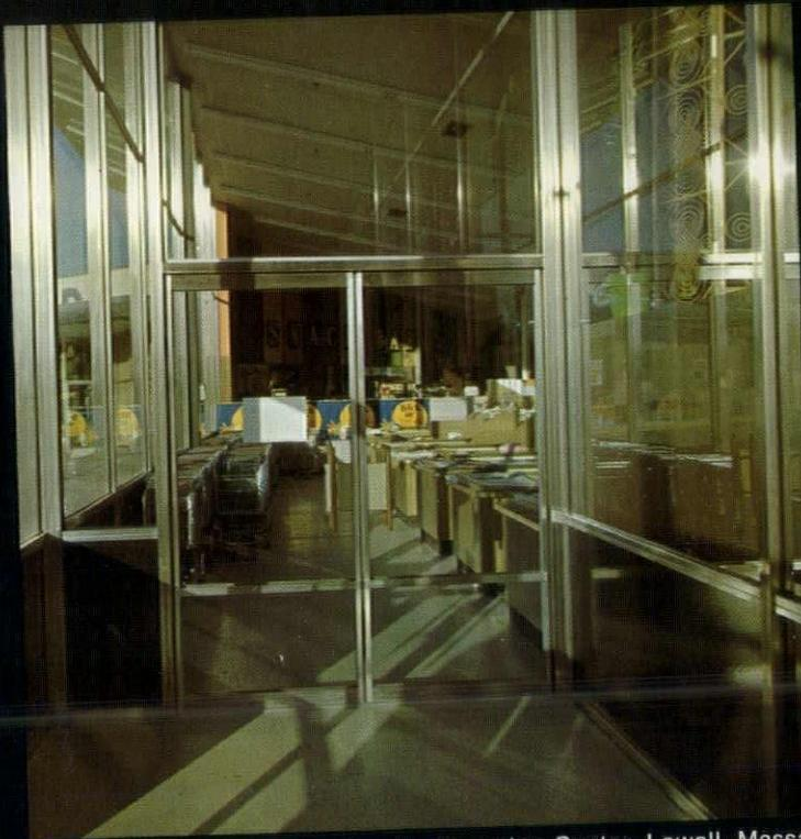
Stuart's Department Store, Sunrise Shopping Center, Lowell, Massachusetts, has 1700 square feet of storefront framed with USS ULTIMET Stainless Steel Wall Framing. It uses 5½-inch mullions for the 19-foot vertical span. The lobby is also enclosed with USS ULTIMET framing. There are eight USS ULTIMET Stainless Steel Narrow Stile Swinging Doors.
