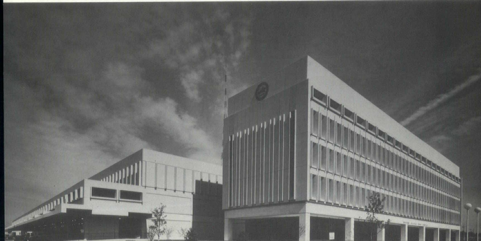
Facade of Price Brothers Corporate Headquarters. Cantilevered construction liberates the fenestration potential of structure.
