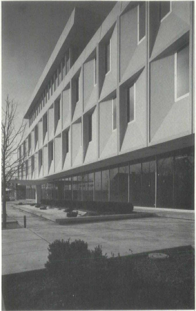
Facade of Price Brothers Corporate Headquarters. Cantilevered construction liberates the fenestration potential of structure.
