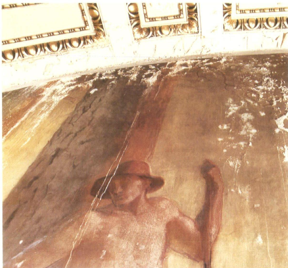
• Science Revealing the Treasures of the Earth, view of surface shows efflorescence and generally deteriorated condition.
