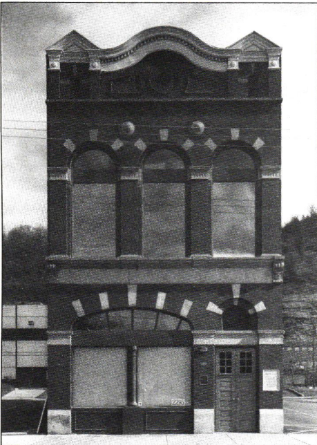
This turn of the century fire station in the Strip District is brought back to life with the help of John Martine, AIA. The building now houses an advertising agency.
