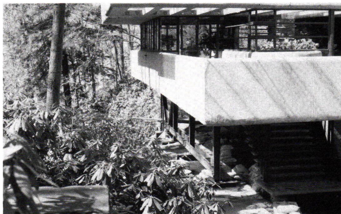
ABOVE: View of Fallingwater from the southeast, showing temporary shoring under the main floor cantilever. Sandbags and concrete blocks dam Bear Run so that steel bases may be grouted into place on the irregular stream bed.
