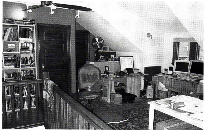
To create an open loft space, they removed walls and ceiling to make a new, higher ceiling that follows rafters.
