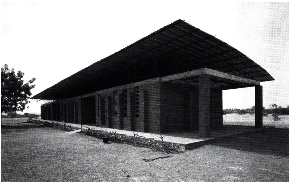
Gando Primary School, Gando Village, Burkina Faso, 1998-2001. A double-roof superstructure overhangs the building, creating shaded areas and preventing the classrooms underneath from gaining heat. Designer – Diébédo Francis Kéré
