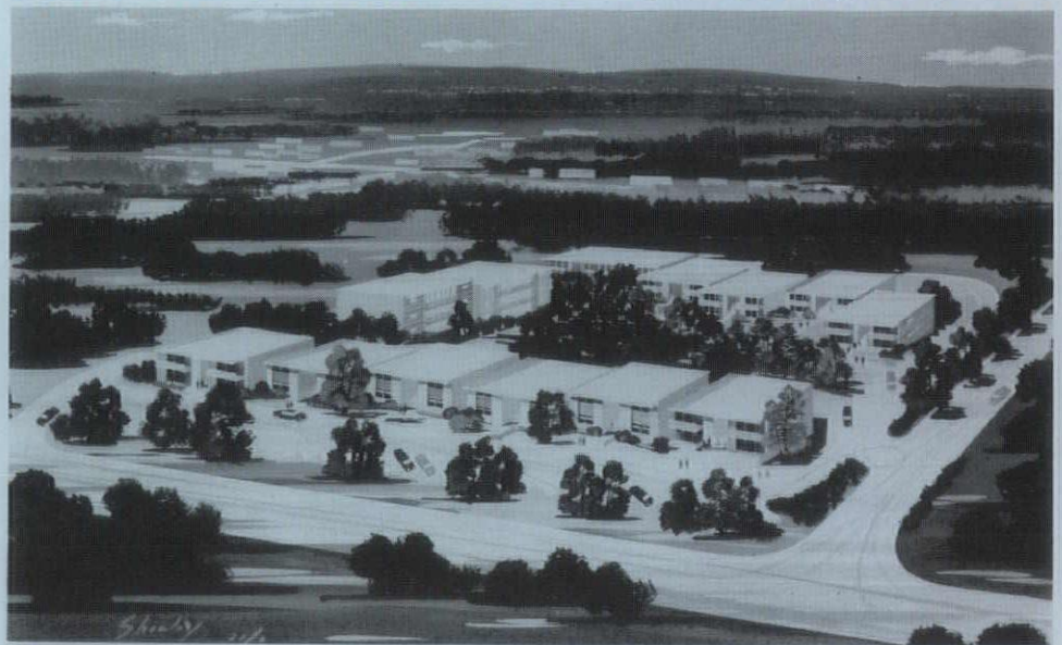
Wheaton House, Wheaton, Md., garden apartments featuring balconies and a landscaped center court. Cohen, Haft and Associates, Architects.
