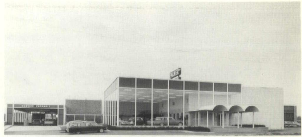
THE PALMER FORD Automobile Dealer Plant, Hyattsville, Md., was commended by the Ford Motor Company for outstanding design. The building is fully air-conditioned and has more than 45,000 square feet of floor area, at a total cost of $350,000. John S. Samperton, Architect.
