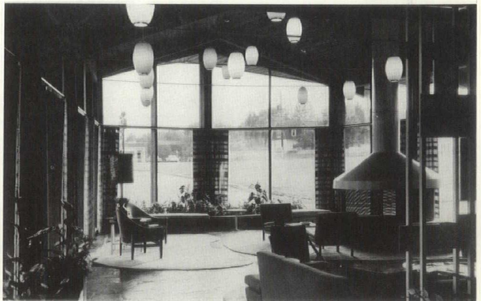
LOBBY OF PARK TOWSON MOTEL
