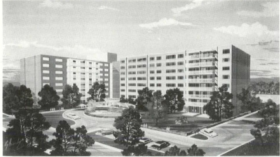
Oglethorpe House, 243 Units, Hyattsville, Md. L. G. Meltzer Associates, Owner
