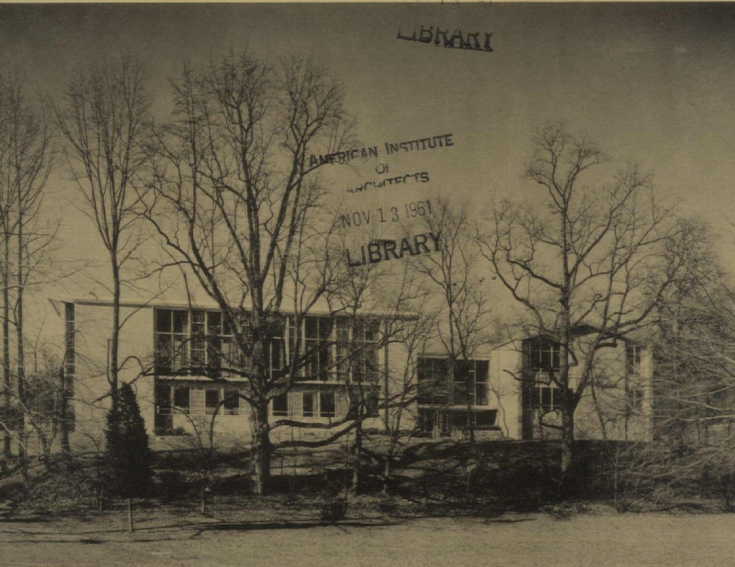
Memorial Evangelical United Brethren Church, Duane & Lawrence, Architects
