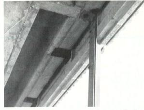
irons—here pictured—stud bolts near the bottom of the panels were secured to stud bolts in sill bottoms. Installation thus was fast, firm, and effective.
