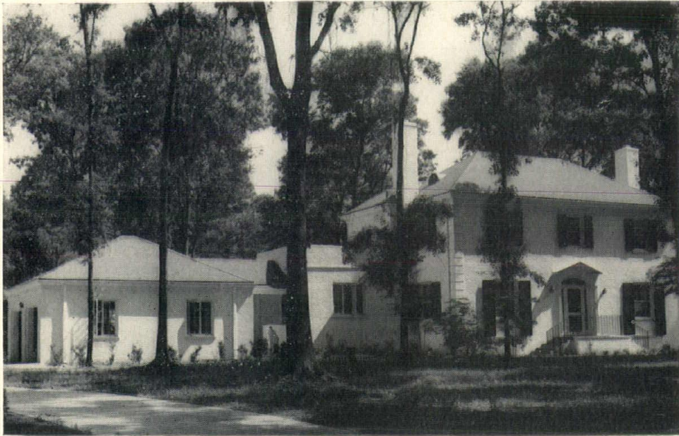
WILLIAM H. COGSWELL RESIDENCE, Charleston Architects: Halsey & Cummings, Charleston General Contractor: C. W. Blanchard, Charleston
