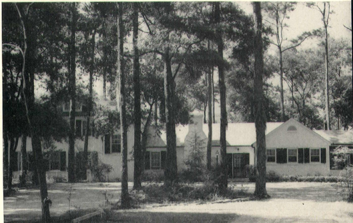
J. U. McKETHAN RESIDENCE, Charleston Architects: Halsey & Cummings, Charleston General Contractor: Dotterer Engineering Company, Charleston AGC
