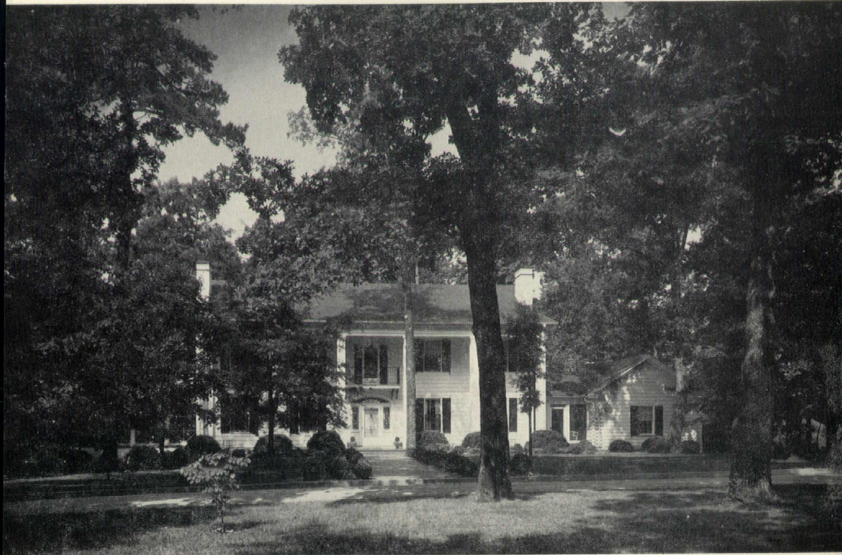
JAMES A. MATTISON RESIDENCE, Belton Architect: William R. Ward, Greenville General Contractor: S. S. Smith, Belton Photo by Gillespie-Cole, Greenville
