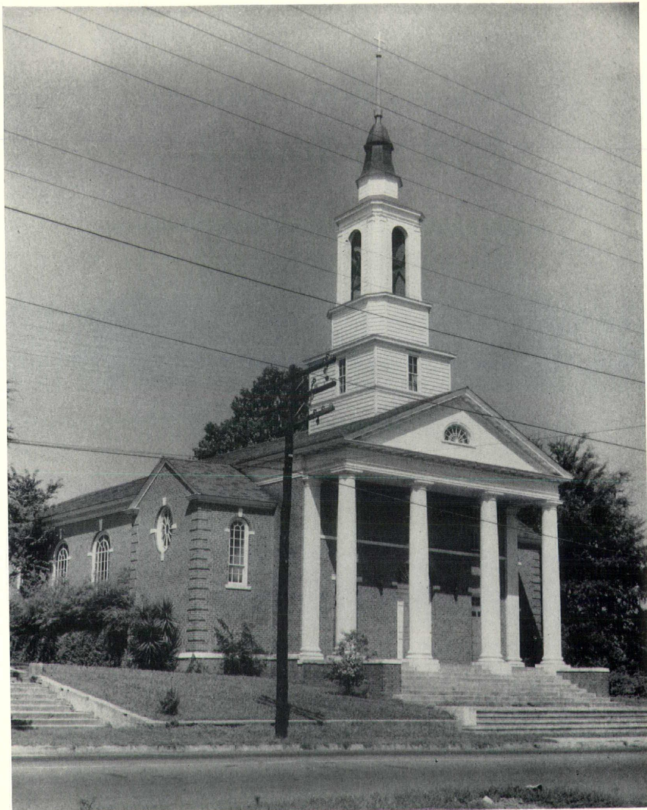
SHILOH BAPTIST CHURCH, Bennettsville Architect: H. D. Harrall, Bennettsville
