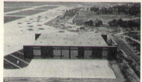
Double Cantilever Maintenance Hangar, Shaw Air Force Base, Sumter, S. C. Architect-Engineer: Kuljian Company, Philadelphia.
