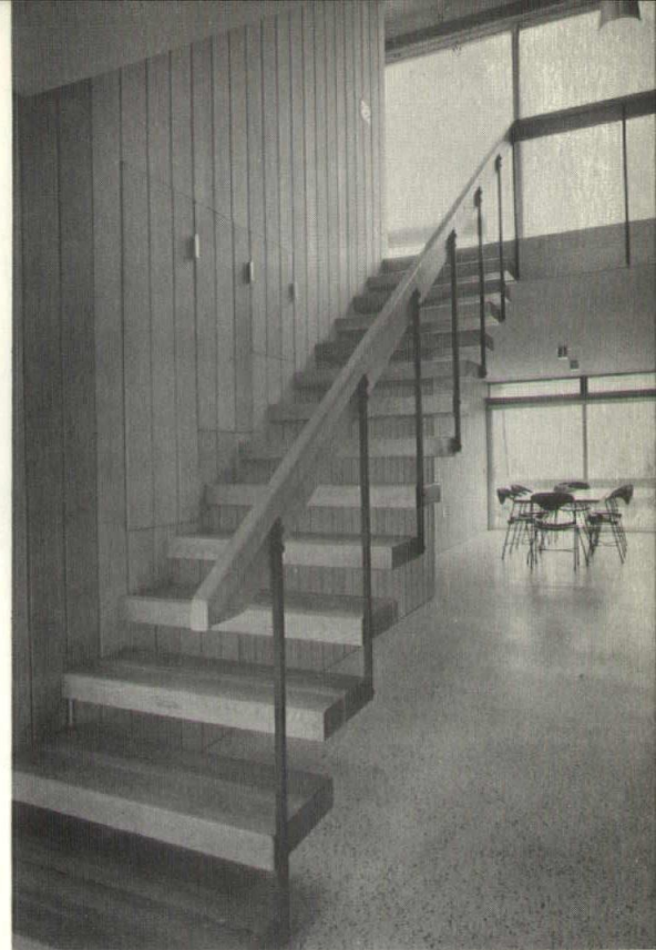
The stair in the entry hall is built by cantilevering the individual 4" x 12" laminated oak treads from the supporting wall, and a concealed storage area.
