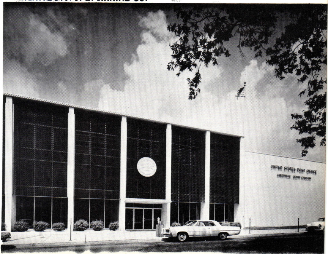
2. UNITED STATES POST OFFICE ARCHITECTS: J. E. SIRRINE CO.
