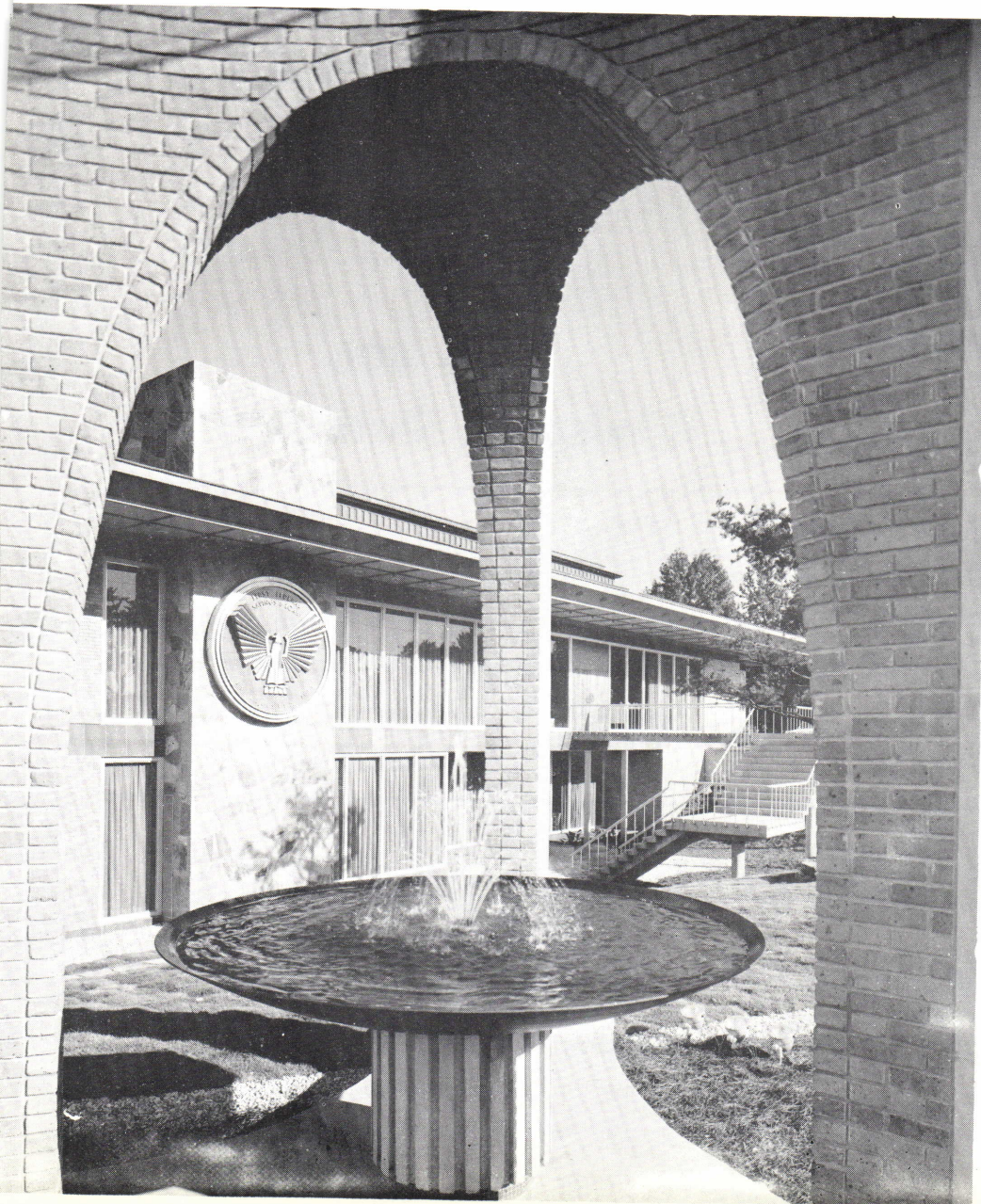
8. WADE HAMPTON OFFICE, FIRST FEDERAL SAVINGS & LOAN ASSOCIATION ARCHITECTS: W. E. FREEMAN, JR. & ASSOCIATES
