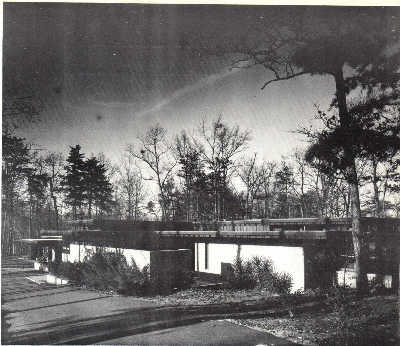
13. PETER SASSO RESIDENCE ARCHITECTS: TARLETON & TANKERSLEY
