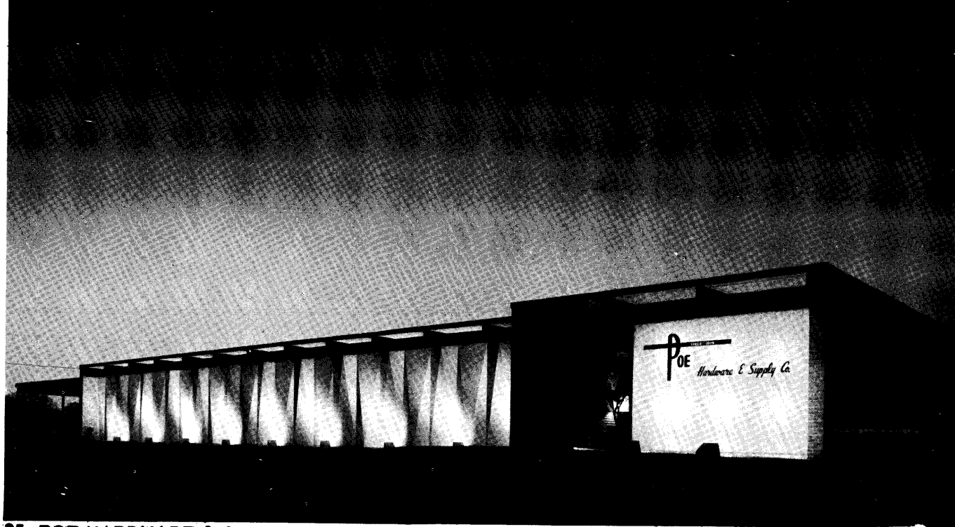
35. POE HARDWARE & SUPPLY COMPANY ARCHITECTS: J. E. SIRRINE CO.
