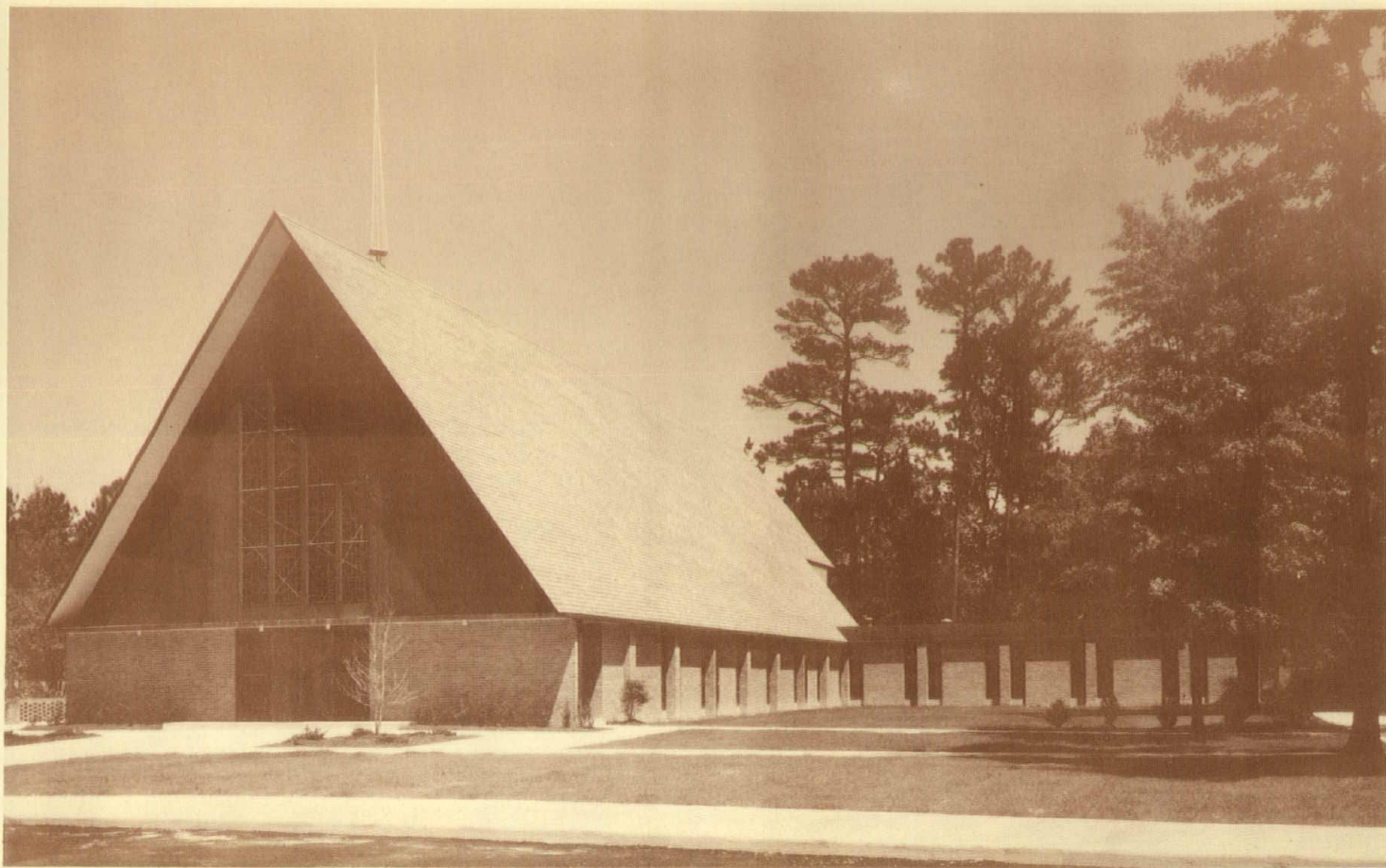
BETHEL METHODIST CHURCH, Columbia Architects: Geiger & Califf Associated Architects
