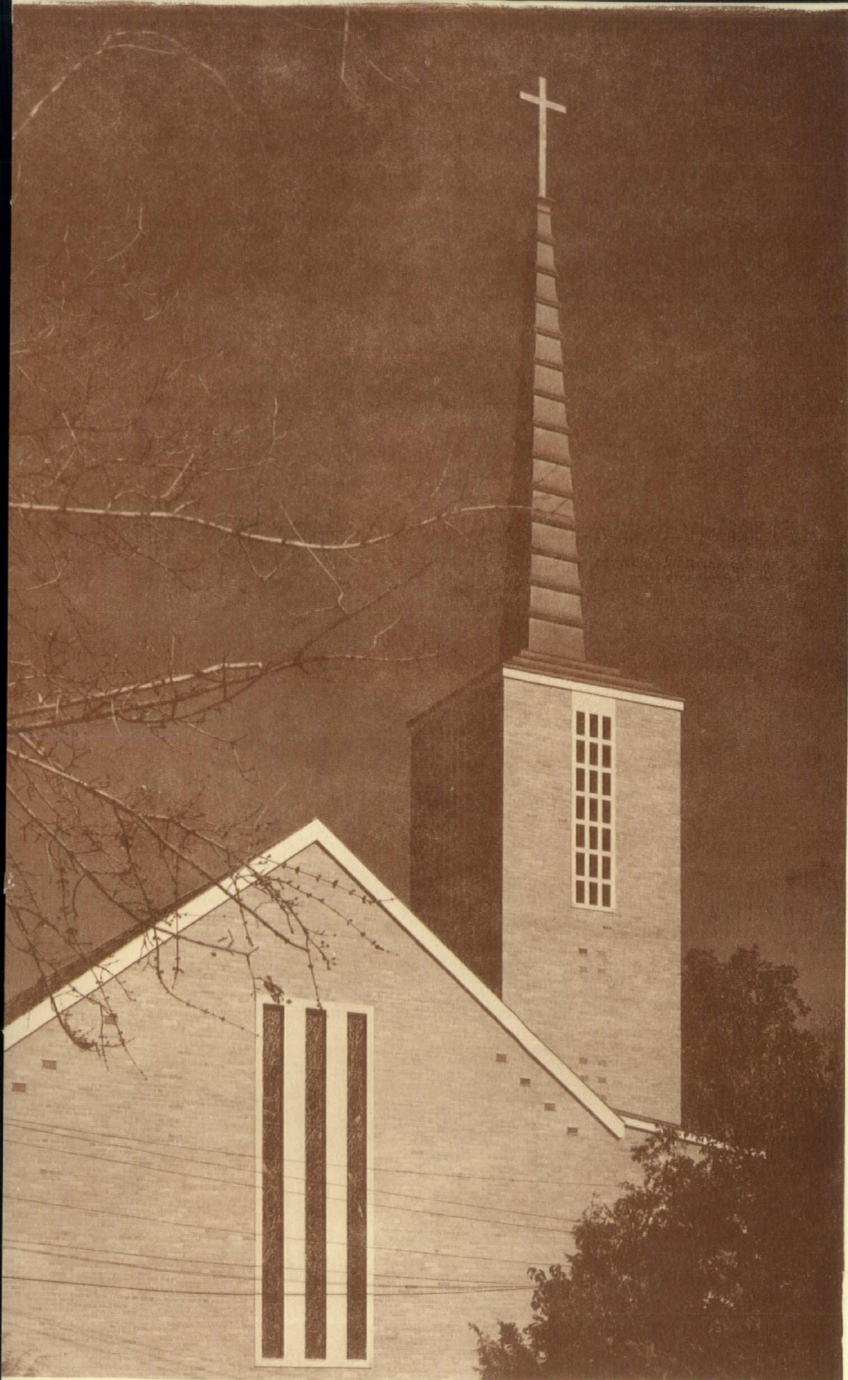
CHESTNUT STREET METHODIST CHURCH Lumberton, N. C. Architect: Charles N. Robinson Lancaster
