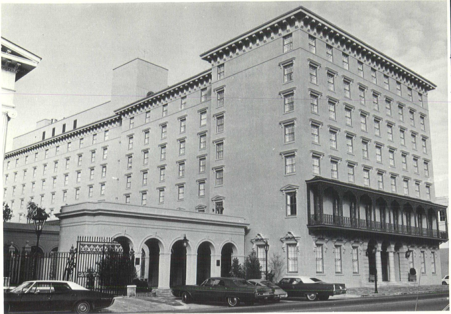
The Mills Hyatt House, Charleston, Curtis & Davis and Simons, Lapham, Mitchell & Small, Architects Ruscon Construction Company, General Contractor
