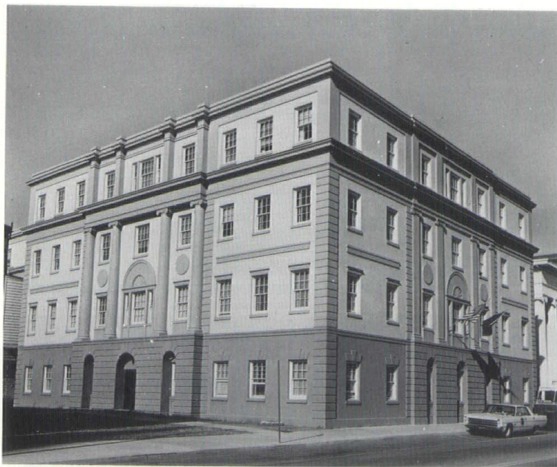
Another new structure in the same block of Meeting Street is Simons, Lapham, Mitchell & Small's County Office Building located on the opposite side of the Ionic columned Hibernian Hall from the Mills Hyatt House. St. Michael's steeple is framed by the scrollwork balcony of the hotel looking down Meeting Street.
