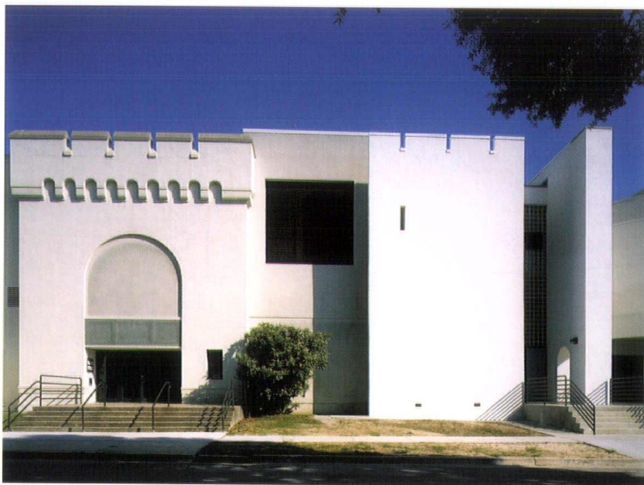
Above: The new Women's Locker facility (right) as it contextually relates to the existing building. Right: The main building entry is through a north-facing glass block wall, 30' high, wedged between two stuccoed planes.
