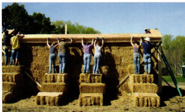
Students placing RBA (roof bearing assembly)
