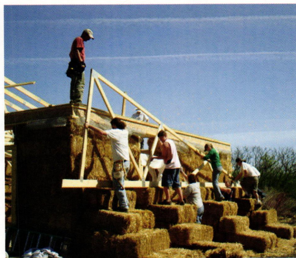
Students placing standard roof trusses
