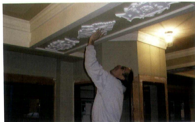
Jastram installed the medallions with recessed screws and prepped them for painting.
