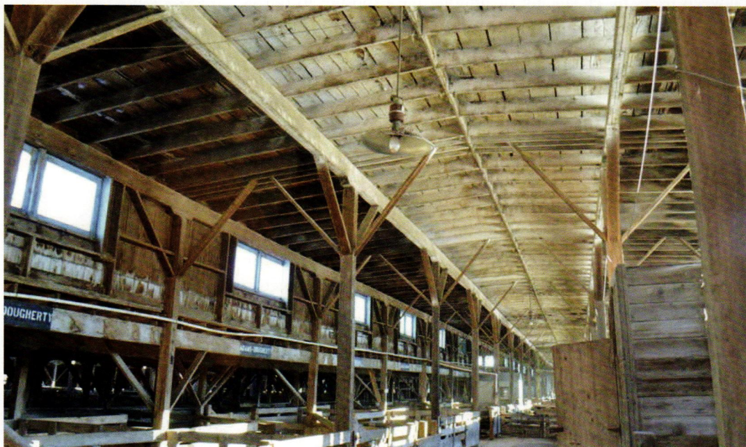
ABOVE: Interior view of timber framing and livestock pens in the stockyards barn. The building was recently removed to make way for site redevelopment. Gate hardware and assorted materials were salvaged, when possible, for integration in future plaza improvements.
