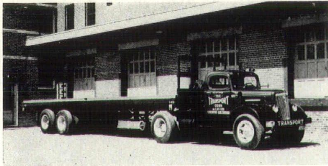
Modern platform trailer used to transport leaf tobacco, machinery, steel and many other general commodities.
