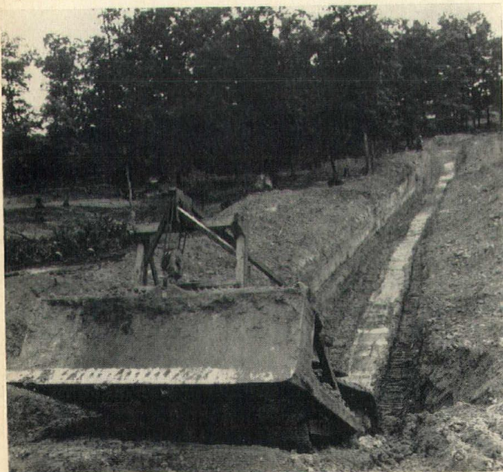
Below, a bulldozer begins the job of replacing an upright silo with a trench silo, which is more efficient and much easier to fill and empty.
