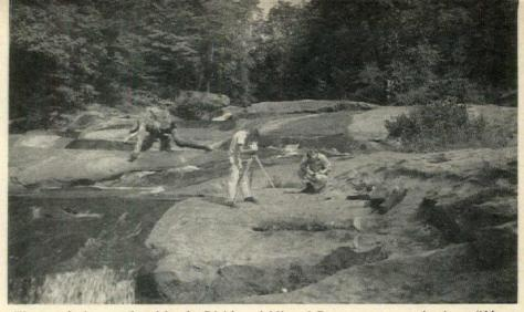
These geologists, employed by the Division of Mineral Resources, are conducting a "Magnetometer" survey, through which information on rock types and mineral deposits is gathered.
