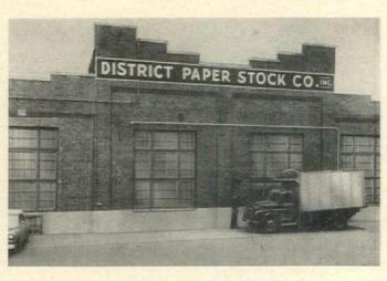
The usual loading from truck to cart is eliminated by giant doors, which permit trucks to back in and unload directly in the plant.
