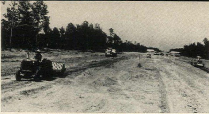
This scene shows grade work on Interstate Route 95 in the vicinity of Dunn, N. C. The finished roadway will contain two 24 foot divided lanes separated by a 36 foot median strip.
