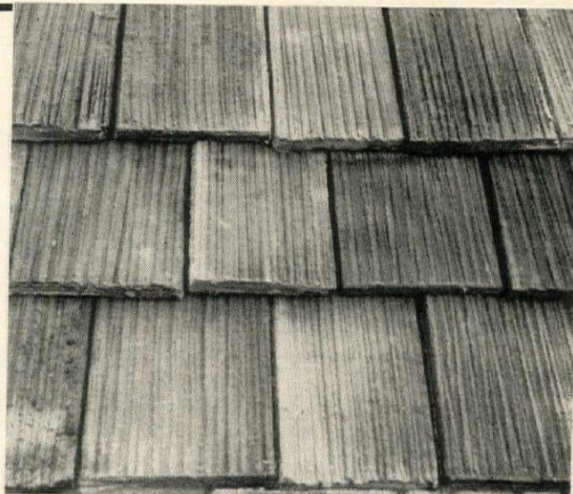
Reproduction of old wood shake roof in concrete.
