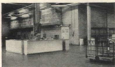
14,407 sq. ft. "Solite refrigerator" main- tains temperatures from 0 to 38° F.
