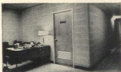
Administrative offices, board room have exposed Solite stack-bond walls.
