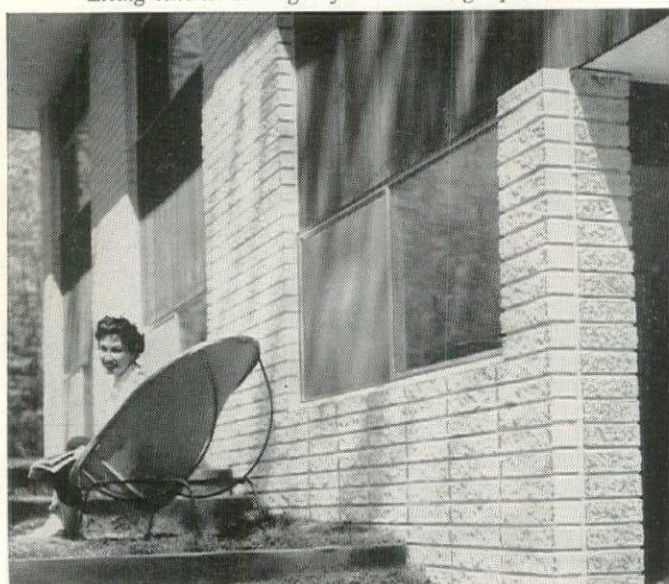
Coarse-textured units in stacked bond for design interest
