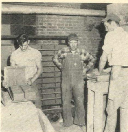
—hand moulding the brick
