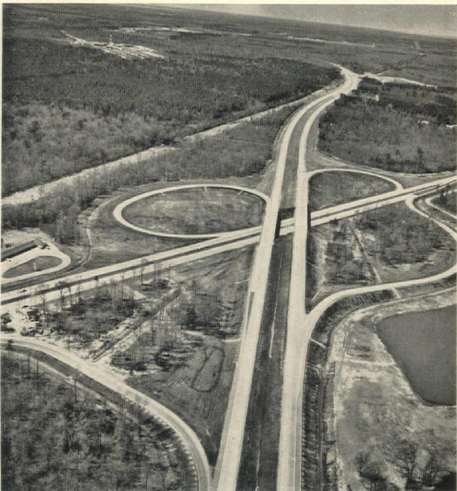
Above, a portion of Route 95 in Hanover County running from near the Henrico County line to Route 54 at Ashland. This section of road, still in the early stages of construction, demonstrates how natural barriers are being maintained when possible to separate opposing traffic lanes. Below, Route 64 in Newport News. Photo shows the interchange with Route 17. This is a part of the Hampton Roads Tunnel approach system. (Photos, courtesy State Highway Department)
