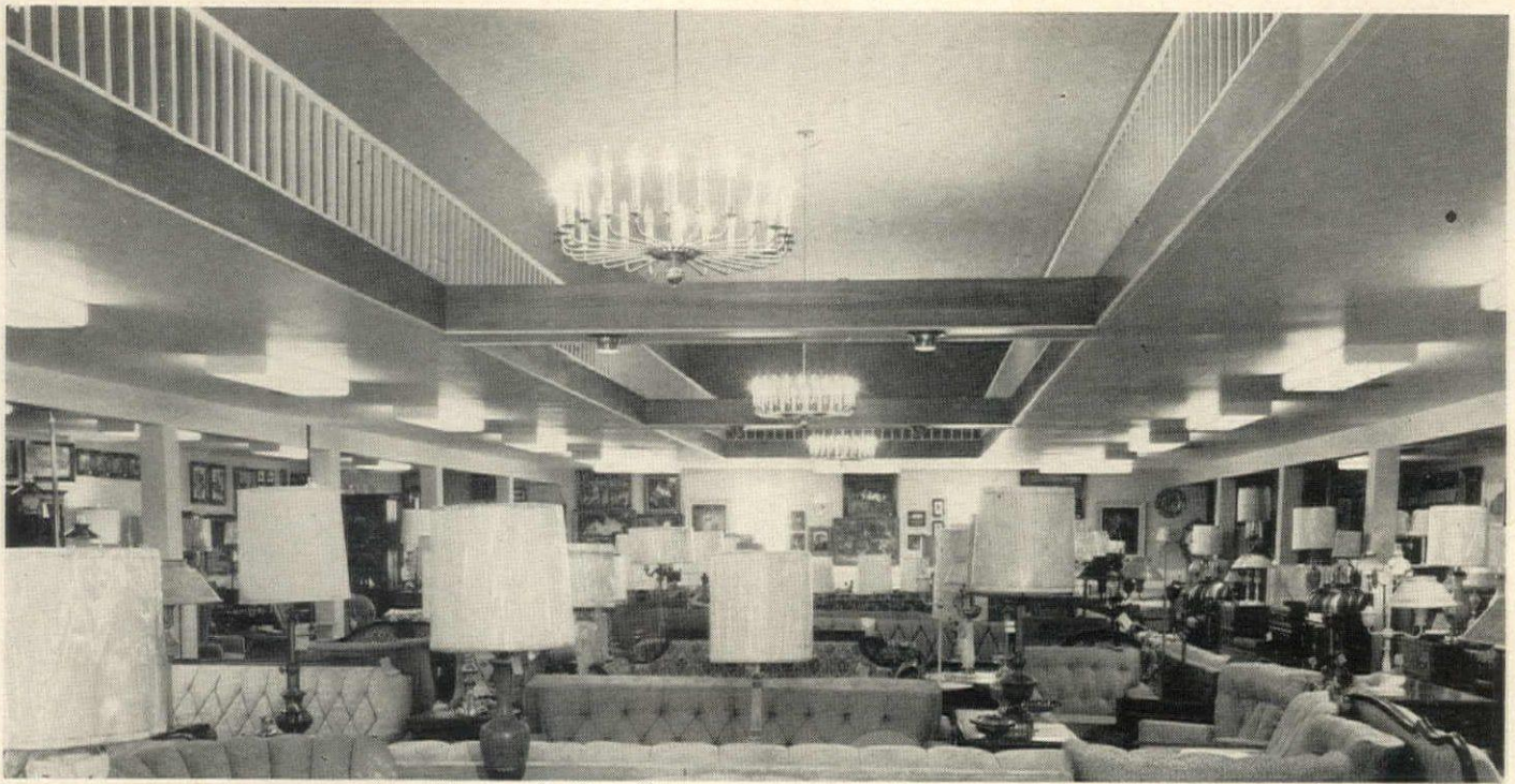
Since the ceiling was only eight feet high, wells were cut in it to give the appearance of a higher ceiling and a balcony was added. Existing rafters were used and trusses made; then at each cross section a brace with turnbuckles was used to keep the building from spreading.
