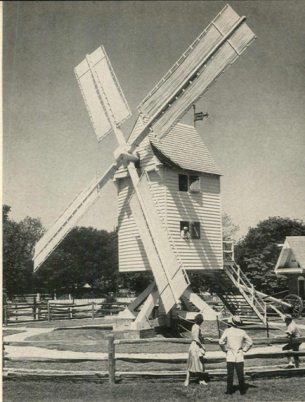
Robertson's Windmill complete, the Storehouse in the background. The mill is known as a Post Mill because the house or "buck," in which the machinery is placed, is supported by a single heavy post braced and supported four ways by quarter bars which are tied at their bearing by heavy sills called cross trees. The buck can be turned to face the wind by the long lever or "tail pole" extending from the buck to the ground at the rear. It is interesting to notice that the steps to the buck must be raised from the ground with a lever before the buck can be rotated.
