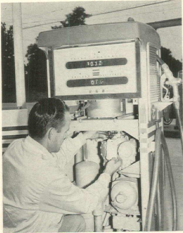
Left: Gas pumps are checked for accuracy and tagged.
