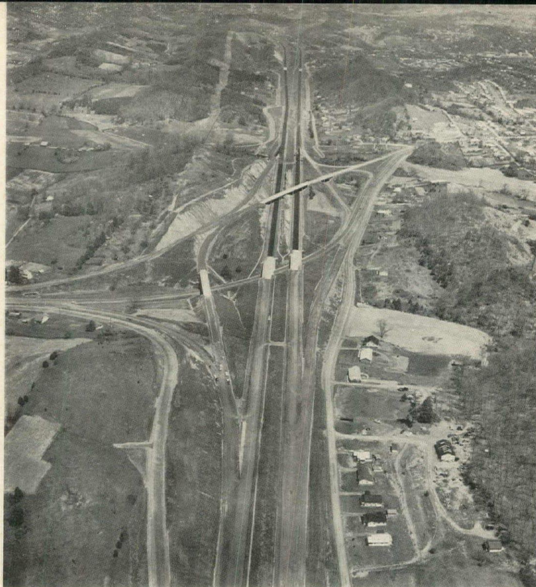
INTERSTATE 95 — ROUTE 301 CONNECTION IN PRINCE GEORGE COUNTY —Below: The recently opened 3.5 mile section of Interstate 95 ties into US Route 301 at this point in Prince George County. This is also an interchange with Route 35. Blythe Brothers Co., Charlotte, N. C., did the grading, bridges and paving under a $2,664,800 contract. This is looking north with the new interstate highway in the upper portion. Route 301 is in the lower left.
