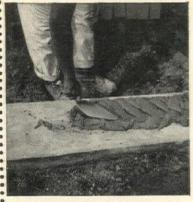
Stays plastic longer. Plenty of time to place and position units carefully—yet mortar made with masonry cement has good body to prevent squeezeout and settlement. Requires less retempering. And its uniform color helps make better looking walls.
