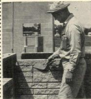
Holds water better for stronger bond. Masonry cement mortar retains high percentage of mixing water—even with porous masonry units. Gives up moisture slowly for better curing, good bond strength. You're sure of tight, water-repellent joints, durable walls. Write for free literature on masonry cement mortars, distributed only in the U.S. and Canada.
