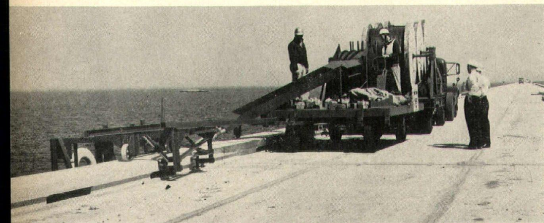
Electrical subcontractor E. C. Ernst devised this cable laying rig, dubbed the "Santa Fe Express" to place power lines in trays mounted on side of trestle.
