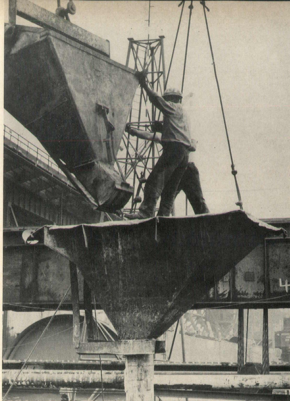
More concrete is piped into pockets between double steel shells to overcome buoyancy of air inside sealed tube. (Photo by Roy)
