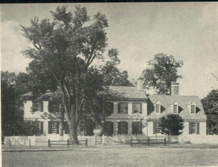
THE PEYTON-RANDOLPH HOUSE, open to the public for the first time, is located on Nicholson Street. Built in three sections, the earliest was the western part, a square house of two stories with central chimneys serving all the fireplaces on both floors, built around 1716. By 1724 a small story-and-a-half house represented by the present easternmost section which was a reconstruction stood upon a neighboring lot. Within a few years these two homes, having come into common ownership, were linked by a two-story middle section. The house is distinguished in a community of many fine homes by its series of paneled rooms. In the ground floor room of the central section, there is a simple grey-veined marble mantelpiece. This mantel and all of the original paneling must date from the first half of the eighteenth century. Occupied by Mrs. F. H. Ball. (Colonial Williamsburg photo)
