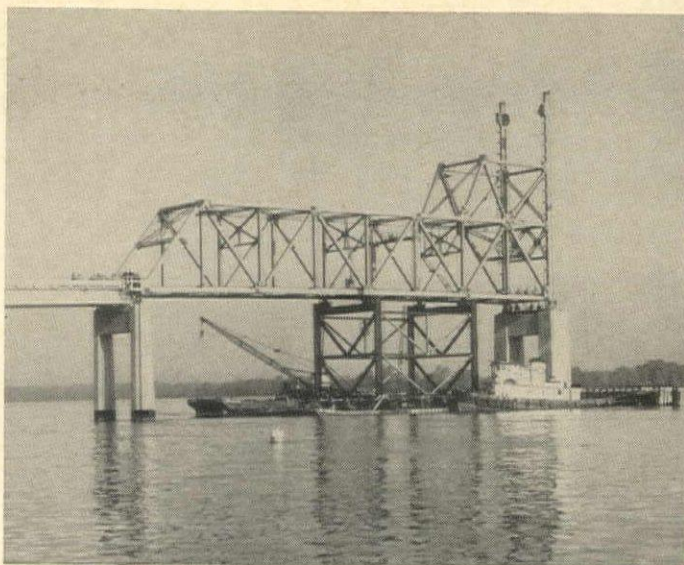
Top photo shows a bridge span, assembled on shore then floated by barge to the site, for the new bridge on Route 156 near Hopewell. Next, a familiar sight to users of Virginia's highways—typical Primary highway construction. Bottom photo shows one of many signs of the times with highway construction moving apace across the reaches of the Old Dominion.
