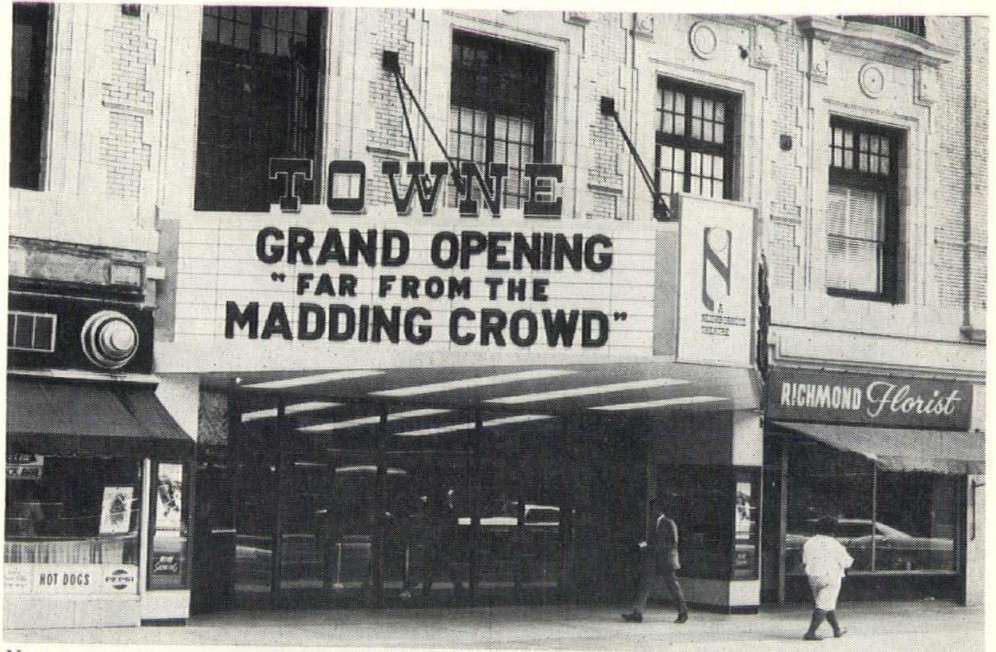
New marquee—entrance & cleaning
