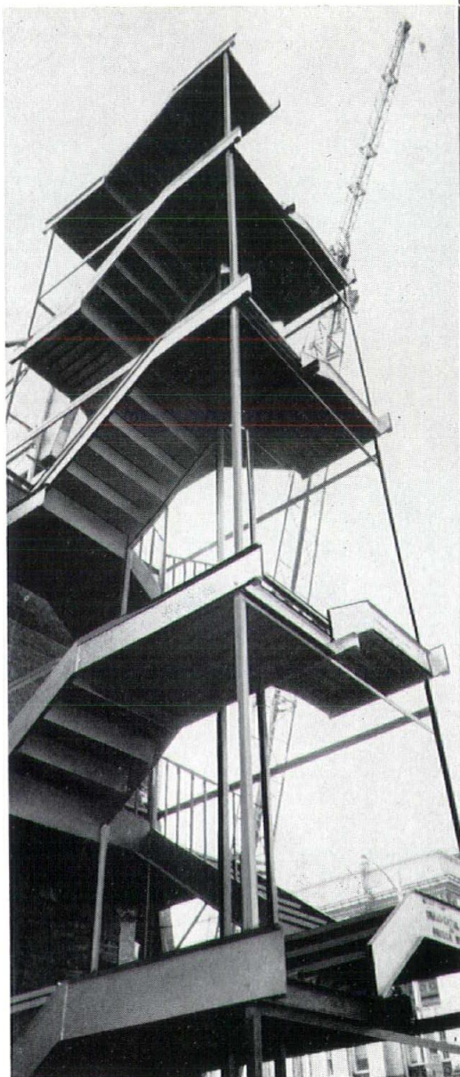
Pre-erected stairway of the new 5-story Southwestern Virginia Savings & Loan Association in downtown Roanoke—produced by Fabricated Metals, Inc.
