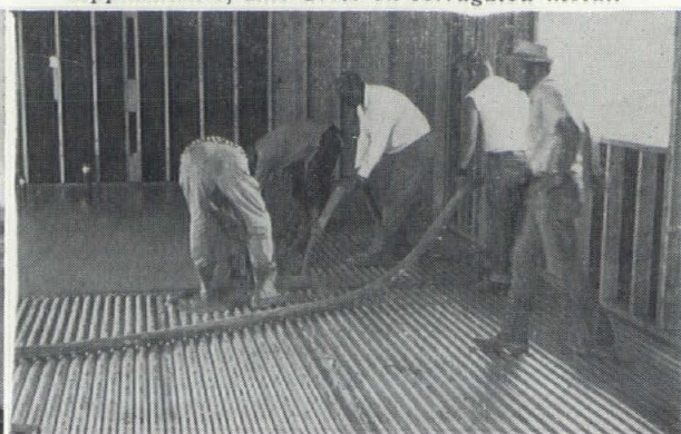
Application of Lite-Crete on corrugated metal.
