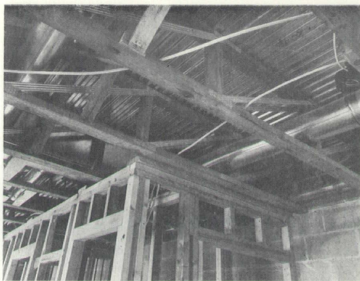
Corrugated metal applied to SPAN JOIST, note ample space for ductwork, plumbing & wiring.
