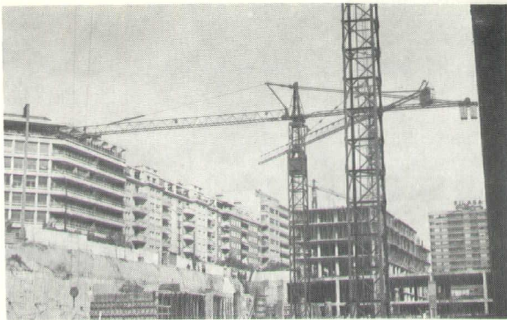
Tower cranes used predominately in Madrid. Virginia Branch Members didn't see a single mobile crane.
