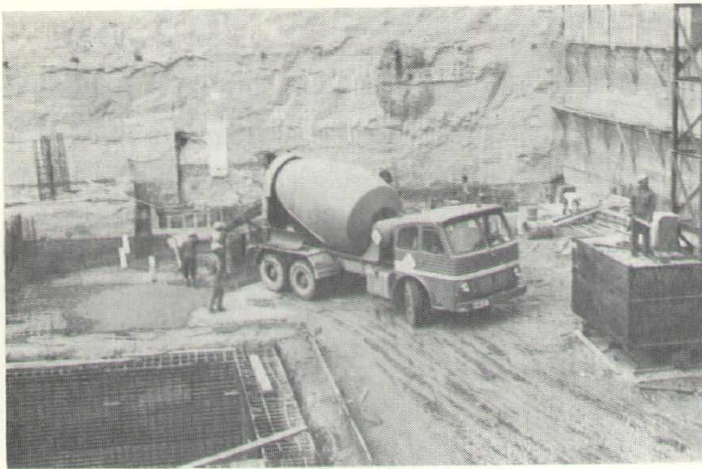
Spanish ready-mix unit delivers concrete to job site.
