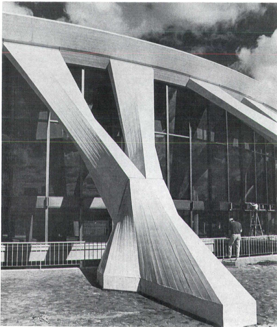
Above, the entrance to the arena is over a bridge spanning a sunken garden. The garage is below the plaza on the right. Below, buttresses are 60 ft. long and weigh 40 tons each. They were poured-in-place using fiberglass molds cast from rough board forms.
