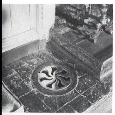
These brass heat registers at Shirley Planta-ion can be closed by a half turn. They were nstalled in 1834, with an iron wood burning tove in the basement supplying the "central eat." The registers were made by slaves on he plantation. (Milwaukee Journal photo)
