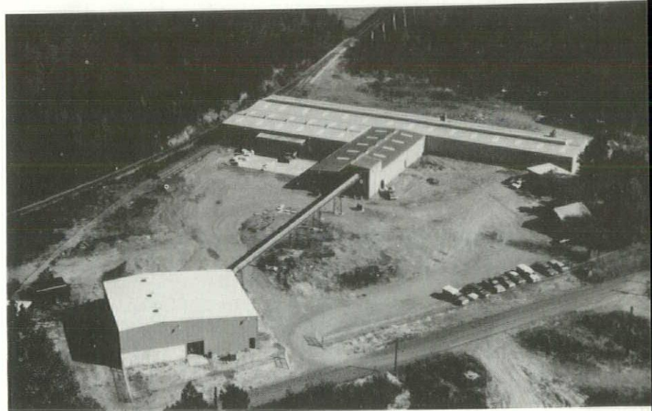
Mid-State's new quarry plant built during 1974 at Mount Gilead, North Carolina. Shale is mined on the property and is ground in the building in the lower left corner and then conveyed to the larger building where the tiles are formed and fired.
