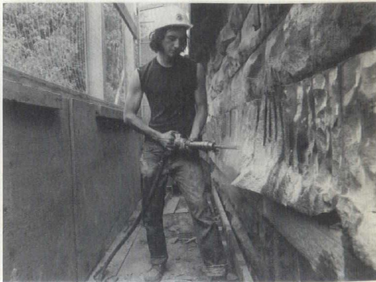
5. Depicts scabbling (roughing, chipping to final surface) in process. (Workman — Richard Chipiwalt)
