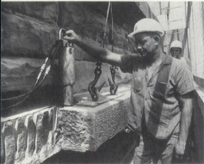
4. Depicts hoist tension by overhead device and hydraulic splitting taking place. (Workmen — Jim Gray foreground, Slocum background)
