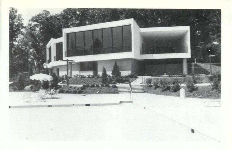
use. The upper level is wood frame on precast concrete plank (required for fire separation). Open and flexible spaces were achieved through the use of long span wood truss joists. The simple shapes are covered with a cementitious coating tinted light beige to contrast with the heavy woods behind.
