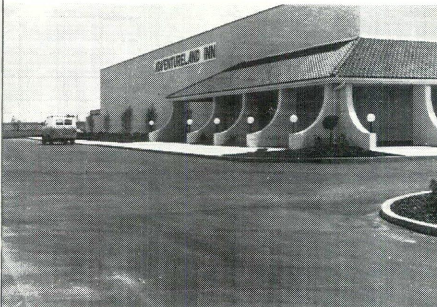
After its temporary service during construction, the layers of asphalt are converted into a permanent surface for the intended use.
