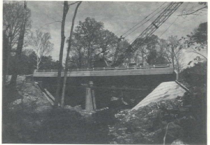
Textured concrete and weathering steel girders help the Forest Hill Avenue bridge blend into the natural surroundings of Forest Hill Park.
