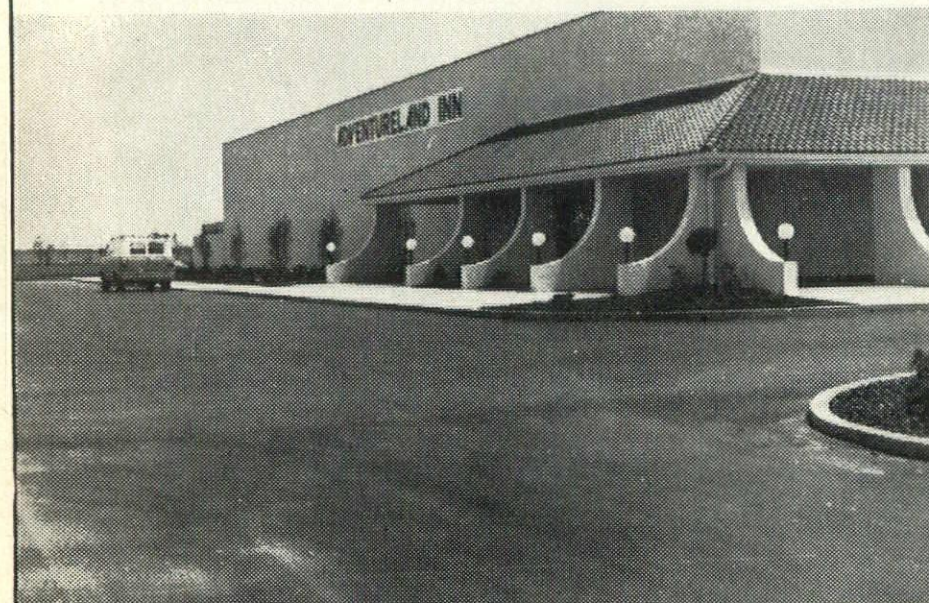
After its temporary service during construction, the layers of asphalt are converted into a permanent surface for the intended use.
