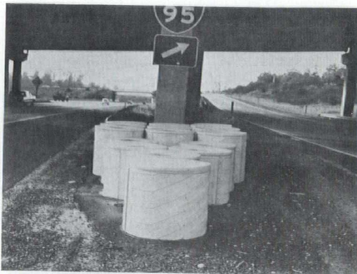
Crash "cushions" such as these sand-filled containers help reduce the severity of vehicles hitting immobile objects such as bridge piers.
