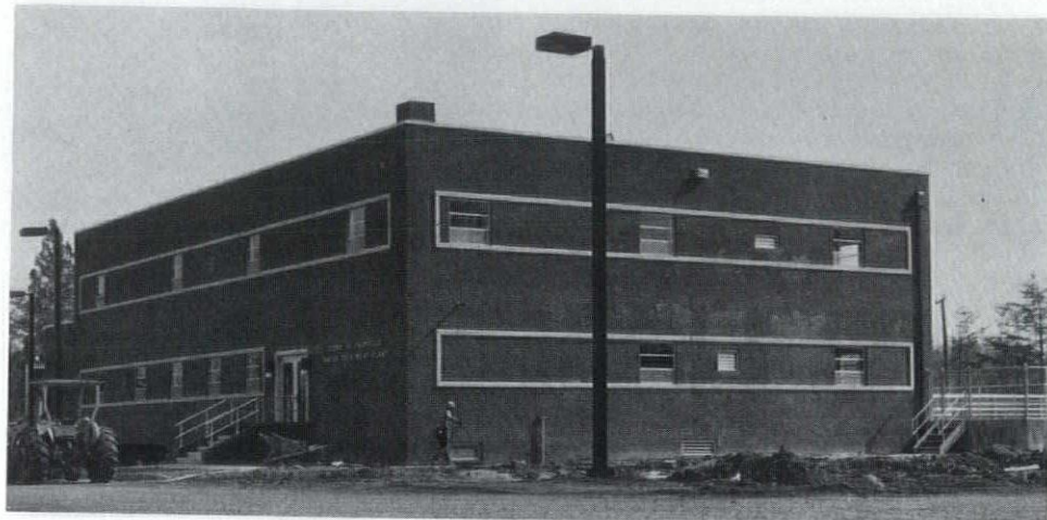
Water Plant Building containing office, laboratory, kitchenette, chlorination facilities, chemical storage and handling facilities, filters, and pumping facilities for the finished water. Portion of Settling Basins is shown at right.
